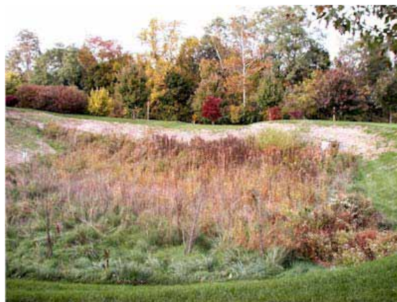
FIGURE 5-43 Dry extended detention pond. SOURCE: PaDEP (2006).
