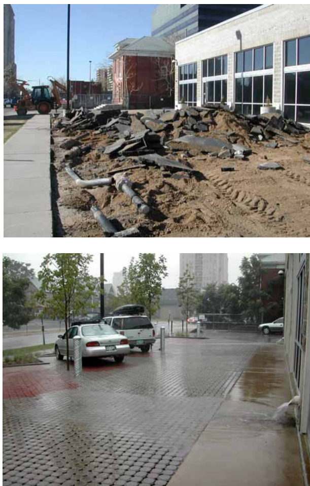
FIGURE 5-32 A small office building conversion at the edge of downtown Denver included the replacement of a portion of the site's parking with modular block porous pavement underlain by an 18-inch layer of crushed rock. Rainfall on the porous pavement and roof runoff for most storm events are contained in the reservoir created by the crushed rock. The pavement infiltrates runoff from most storm events for one-third of the impervious area on the half-acre site. SOURCE: Courtesy of Wenk Associates.
