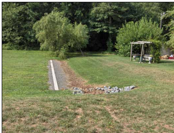
FIGURE 5-11 Level spreader. SOURCE: Robert Traver, Villanova University.
