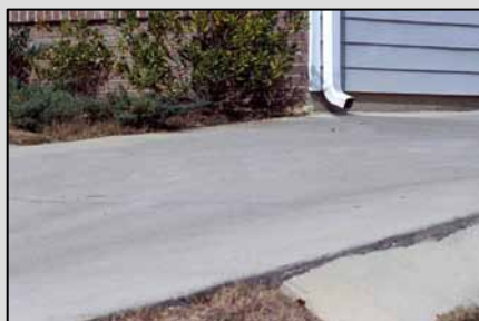
A directly connected roof drain
