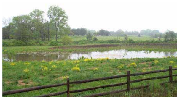
FIGURE 5-42 Wet pond. SOURCE: PaDEP (2006).
