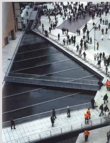
FIGURE 5-59 As shown to the left and below, stormwater is collected and stored on-site in a series of vaults. Water is circulated through a series of biofiltration areas and used for toilets and other mechanical systems in the building complex. Large storms overflow into an adjacent canal. SOURCE: Reprinted, with permission, from Herbert Dreiseitl, Dieter Grau (2001). Copyright 2001 by Birkhäuser Publishing Ltd.
