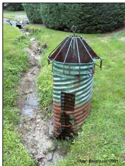
FIGURE 5-50 Rusty outlet structure. SOURCE: Reprinted, with permission, from Emerson. Copyright by Clay Emerson.
