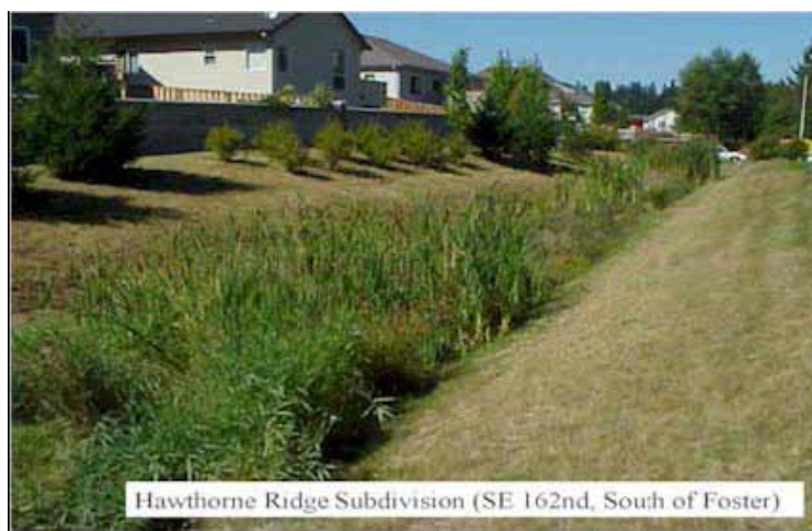
FIGURE 5-16 Vegetated swale. SOURCE: PaDEP (2006).
